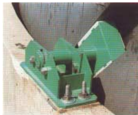
Non-rotating block assembly for a spirally guided Gasholder.
