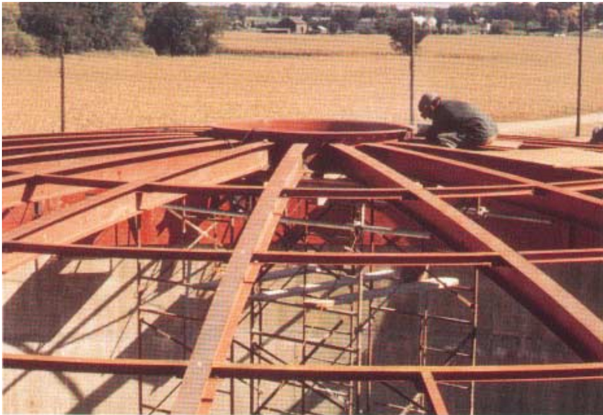
Fixed Cover under erection prior to roof placement.
