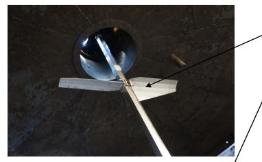
• One set of 2 impellers, mounted near the top of the digester
