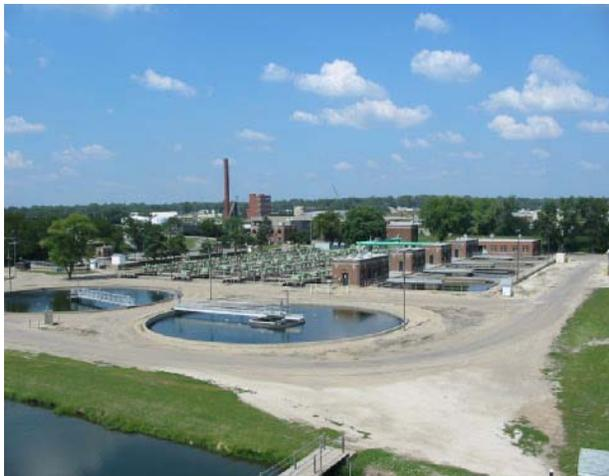
The treatment plant serving the City of Peoria, shown at left, is designed to treat an average flow of 37 million gallons of wastewater every day. The plant was originally built as an activated sludge plant and eighty four (84) RBCs were added later, as a second stage, to remove ammonia, demonstrating the use of RBCs as a cost effective method of nutrient removal. An aerial view of the RBCs follows.
