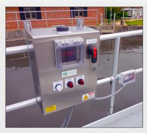
Instrument Panel is mounted on the handrail and allows easier viewing of the digital readout at or near the drive unit.
