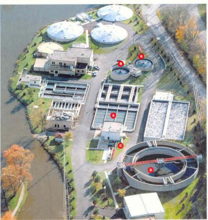
The City's 4.2 mgd wastewater treatment plant is located on the Fox River about 40 miles west of Chicago. Four(4) Walker Process Hydrolink Rectangular Primary Clarifiers were added in 2002 as part of an overall upgrade that increased capacity from 3.5 to 4.2 mgd. Other Walker equipment at this facility include:
